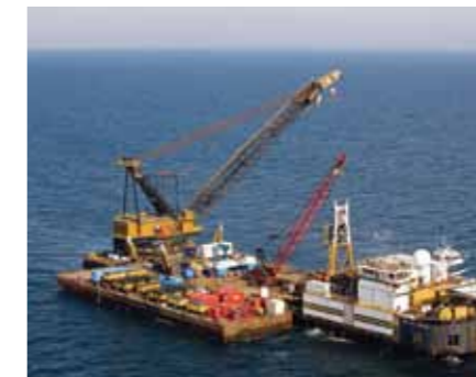
Atlas Copco industrial rental compressors in action during pipeline pre-commissioning in deep water.
